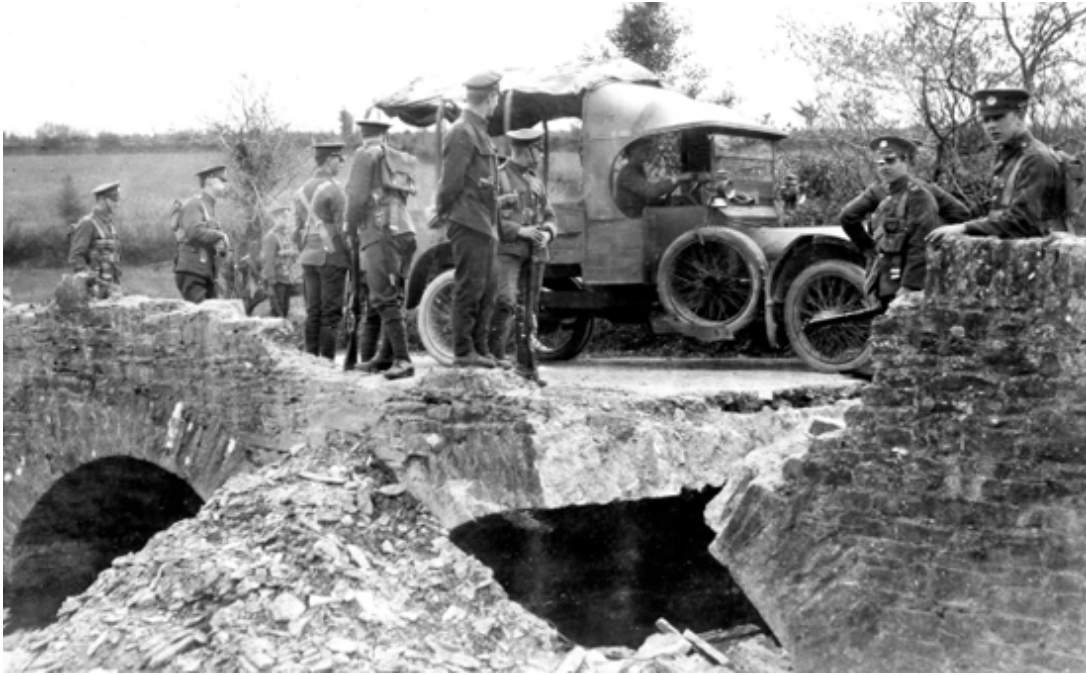
Bridge near Kinsale blown up by the I.R.A.
