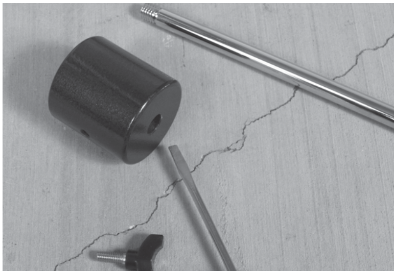
Figure 52-14 Prepare the counterweight.
