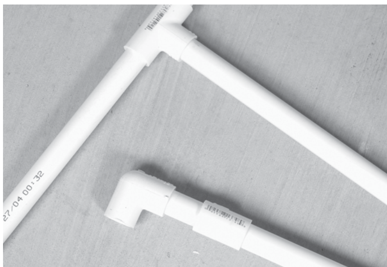
Figure 86-3 Small extensions can be made from leftover pieces of tubing.
