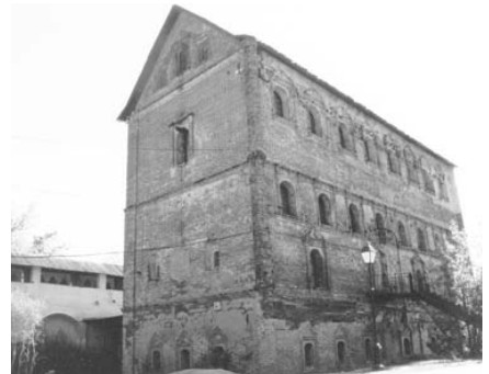
Fig. 14.232. Old building at the New Simonov Monastery in Moscow. General view. Photograph taken in 2000.
