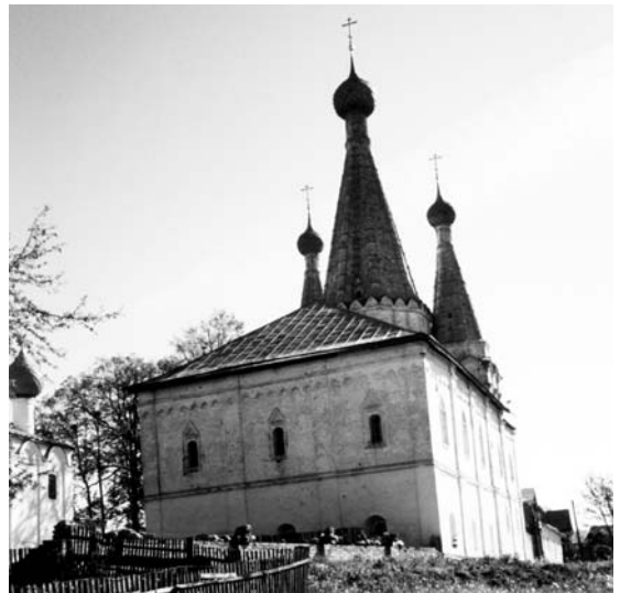
Fig. 14.223. Church of Metropolitan Alexei in Ouglich. Western view. Photograph taken in 2000.
