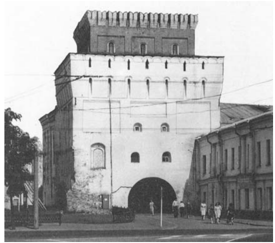
Fig. 14.2. The Vlassyevskaya, or Znamenskaya tower that had formerly been part of Yaroslavl’s sturdy fortifications, destroyed in the Novgorod pogrom (according to our reconstruction). A view from the west. Modern photograph. Reproduced in accordance with [996], page 73. In the left corner of the Znamenskaya Tower one can clearly see the remnants of a brick wall, which had once stood adjacent to the tower. The wall was destroyed – there is nothing left but uneven marks.
