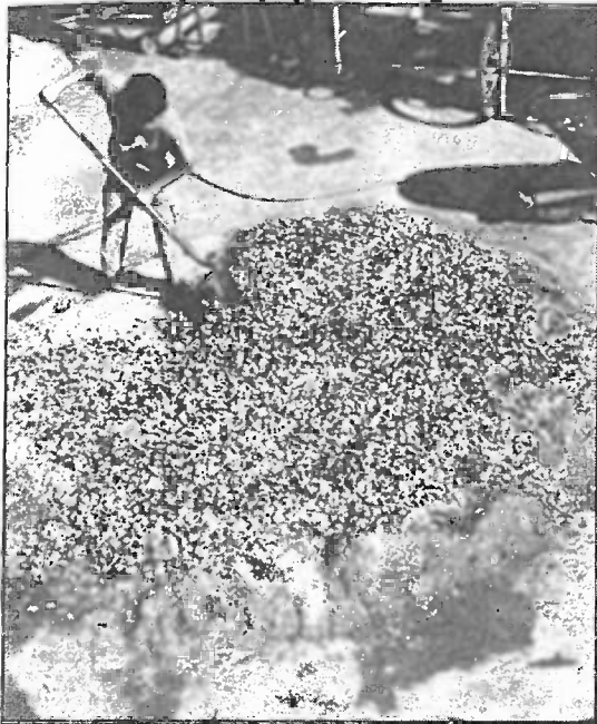
Figure 132. Adding 2-3" diameter wood chips on top which builds the matrix.
