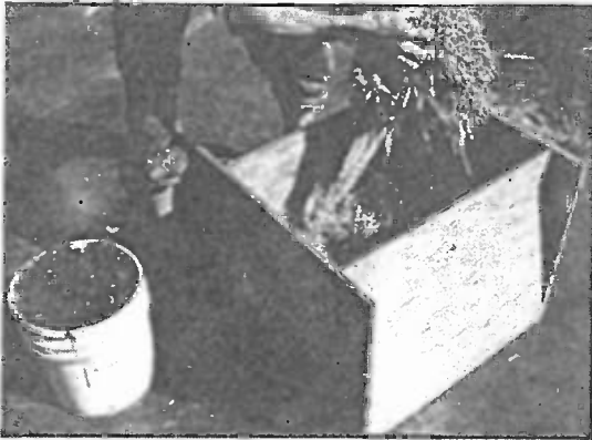
Figure 303. Soaked straw is thrown into a tapering, trapezoid-shaped form.
