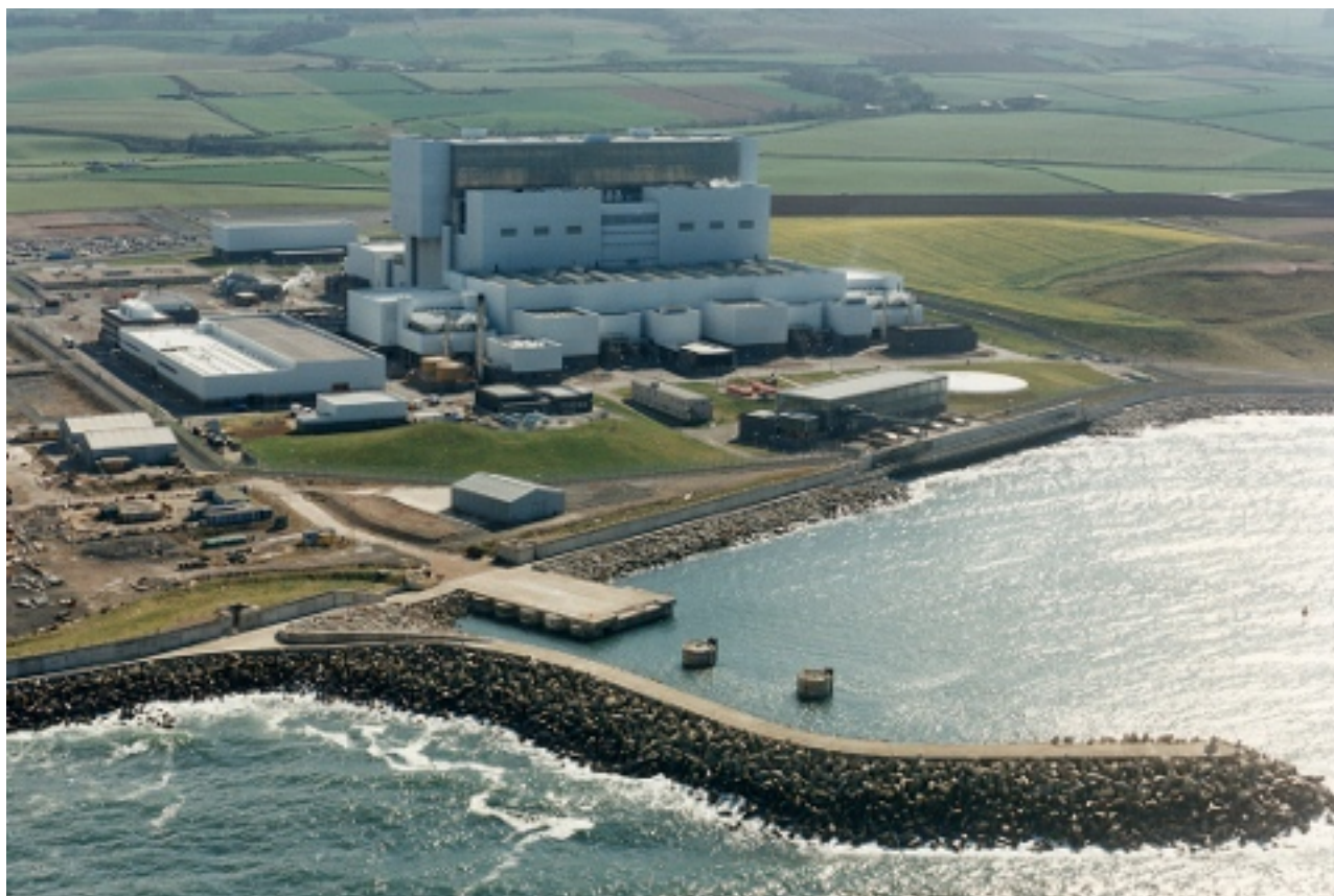
Torness nuclear power station
