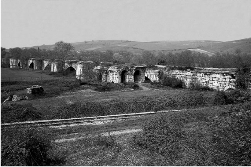
Figure 9.4 Sangarius bridge, c. AD 560.
